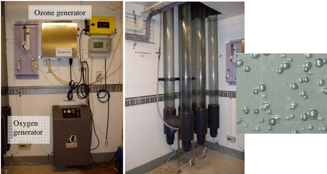
**Figure 8.** The generators, the six ozonation columns and ozone bubbles.
