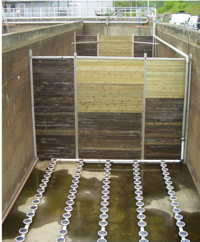
**Figure 5** An empty tank in Sternö WWTP with fine bubble diffused aeration.
