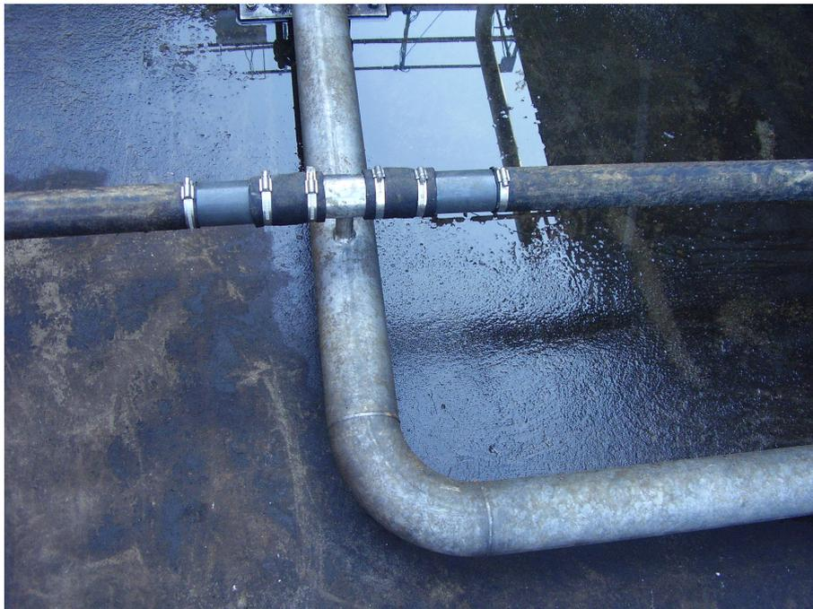
**Figure 7** Fine bubble tube diffusers of unknown brand in (empty) basin in Sternö WWTP. The large pipe at the bottom is the air piping and the small pipe is the diffuser.
