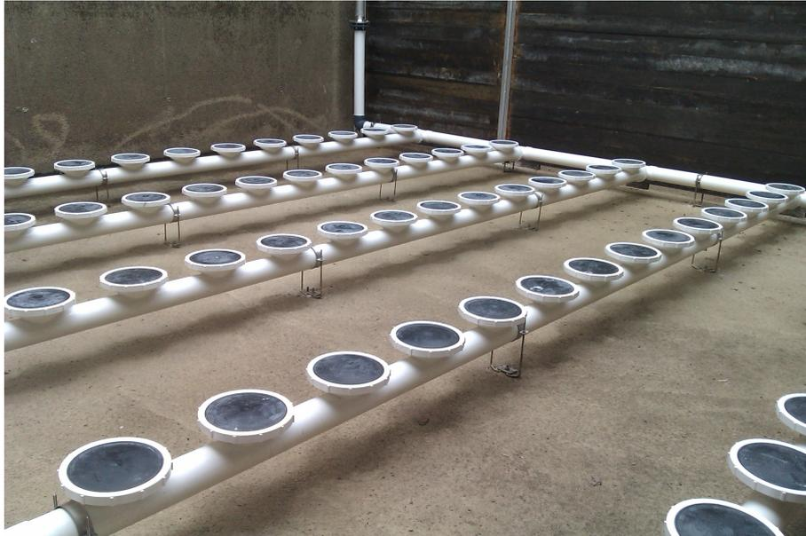
**Figure 8** Newly installed Sanitaire fine bubble disc diffusers in (empty) basin in Sternö WWTP.
