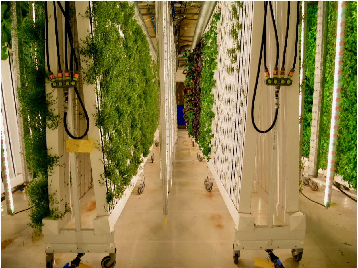
Figure 7 Main growing room with growing towers standing on carts. In the middle of the two carts are ventilation pipes and LED panels. Own picture, SweGreen farm.
