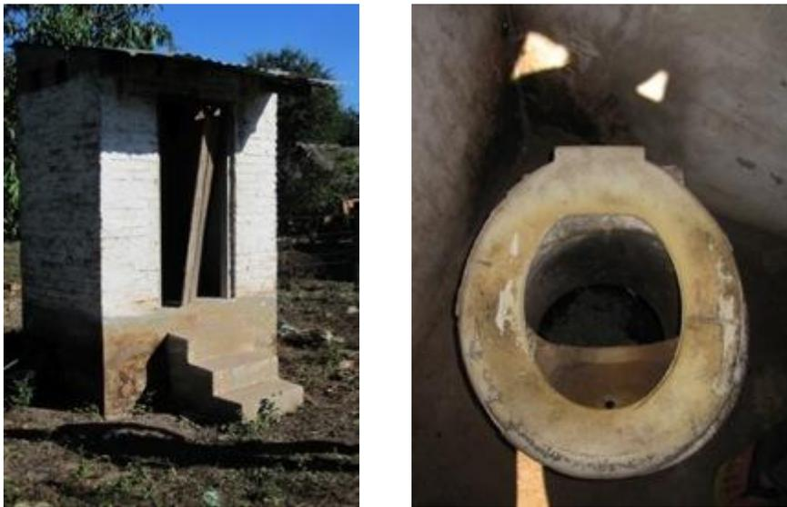
*Figure 36. Toilets in Saveedra lacking in maintenance. Left photo shows toilet with broken door and right photo shows a dirty, broken toilet ring.*
