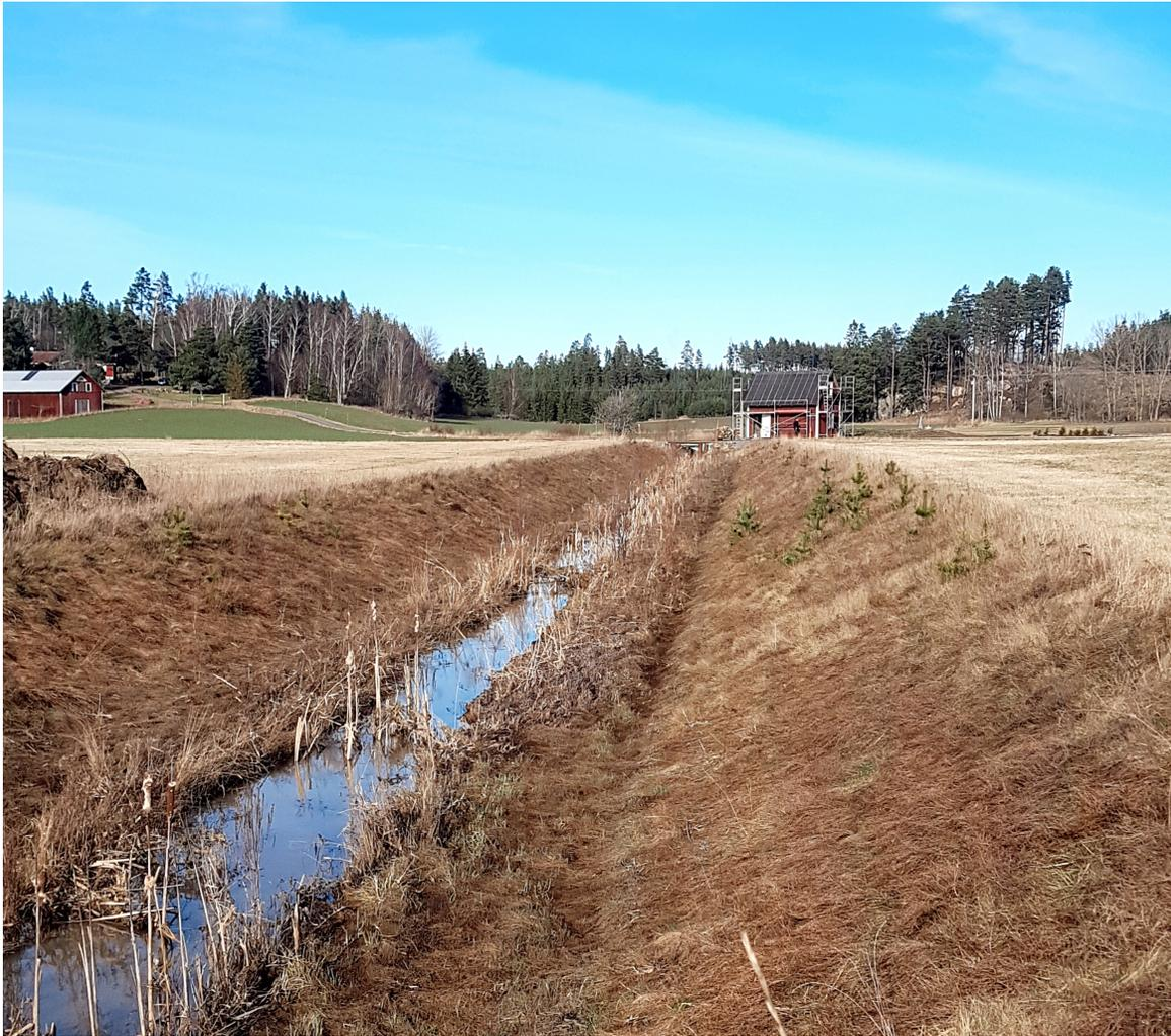
Figure 1: A two-stage ditch in field, located in Sweden. During low water flows, the water is kept in the main channel. During high water flows, the water floods over the terraces. Picture source: (Englund, 2020).
