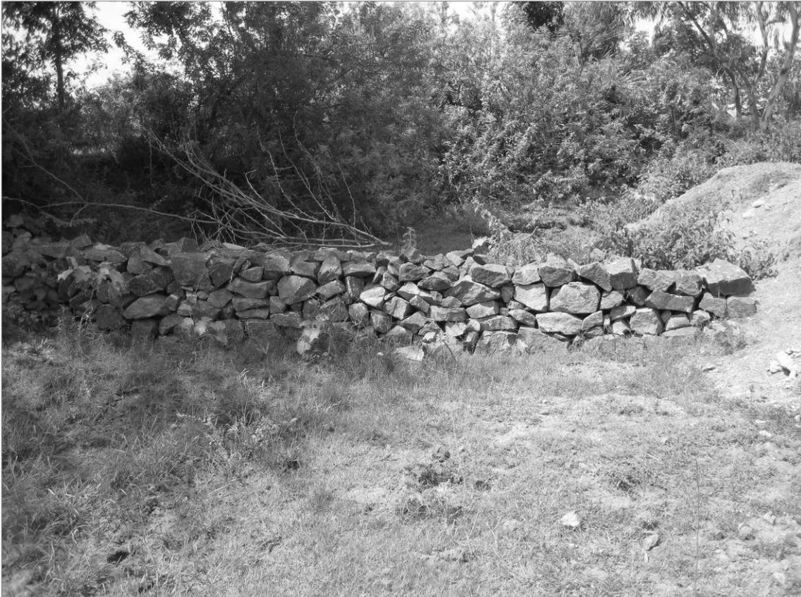
**Figure 3** Gully plug in Arapedu.
