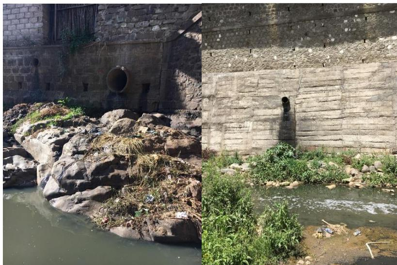
*Figure 15. Outlet observed in the Kebena river, likely part of stormwater system.*
