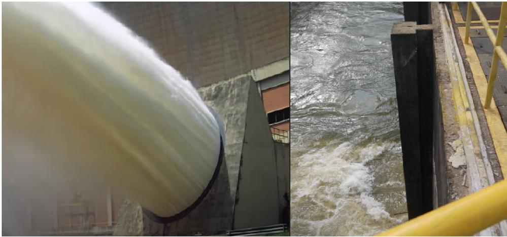
Figure 2. To the left its the outlet for Funil’s degassing process during high water levels and the picture to the right is the outlet for Chapeu D’Uv’as degassing process during high water levels (Wilson 2020).
