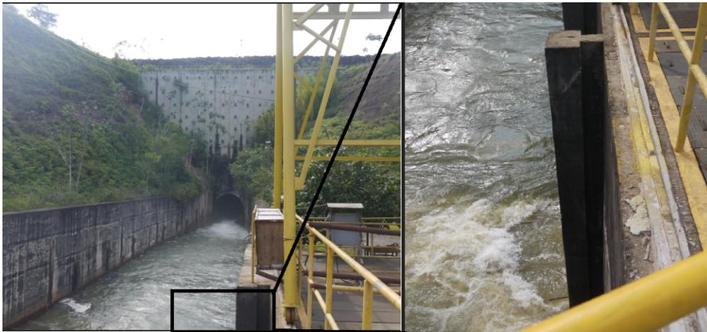
Figure 7. The outlet of Chapeu D'Uvas, the picture to the left shows a outflow of surface water from the spillway that is activated when the reservoir is at max capacity. The right picture shows the outflow from the water intake at 35 meters depth
