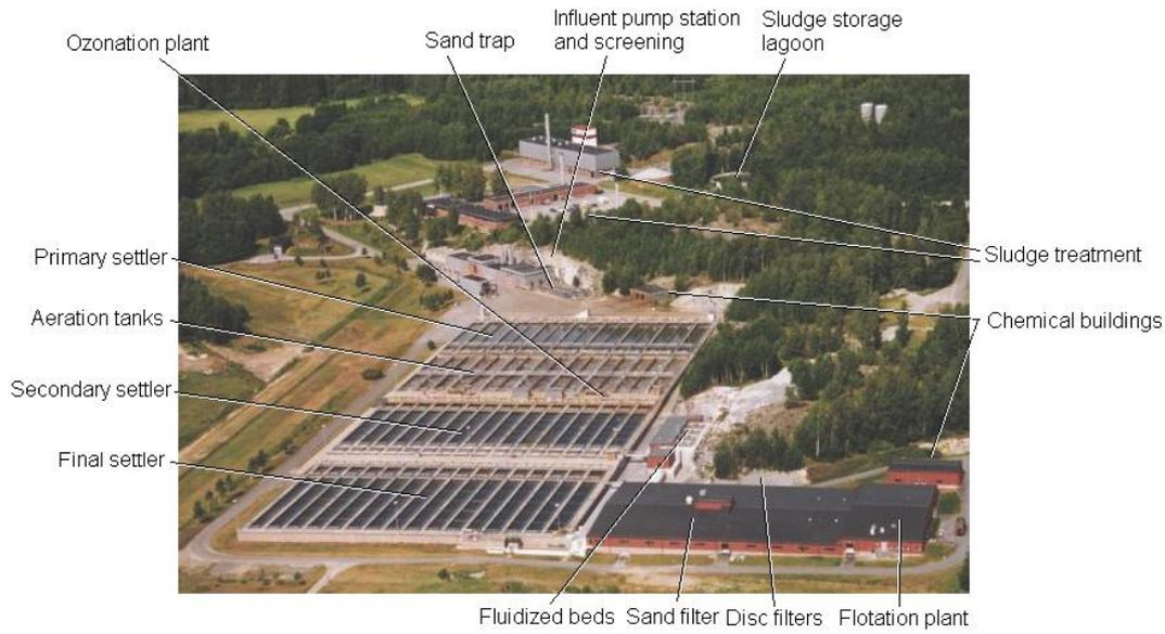
*Figure 9.* Overview of Himmerfjärden WWTP. The capacity of the biological and chemical unit is  $3.9 \text{ m}^3 \text{ s}^{-1}$  and towards the mechanical unit  $5.2 \text{ m}^3 \text{ s}^{-1}$ .
