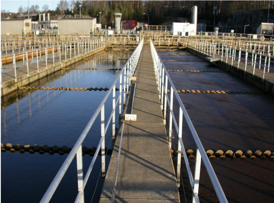
*Figure 12.* The experimental and control line. The surface of the control line (right) is covered with sludge, and the experimental line (left) has a clear surface of water.
