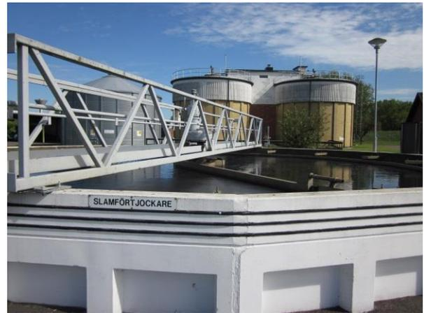
**Figure 3** The image to the left show the gravimetric sludge thickening process and the image to the right show how a gravimetric sludge thickening facility can look like in reality (Kävlinge kommun, 2015).
