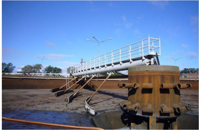
The wastewater enters the PST in the middle of the tank. It is discharged tangentially through numerous pipes, 1 and 1.8 meters below the surface (Figure 6).
