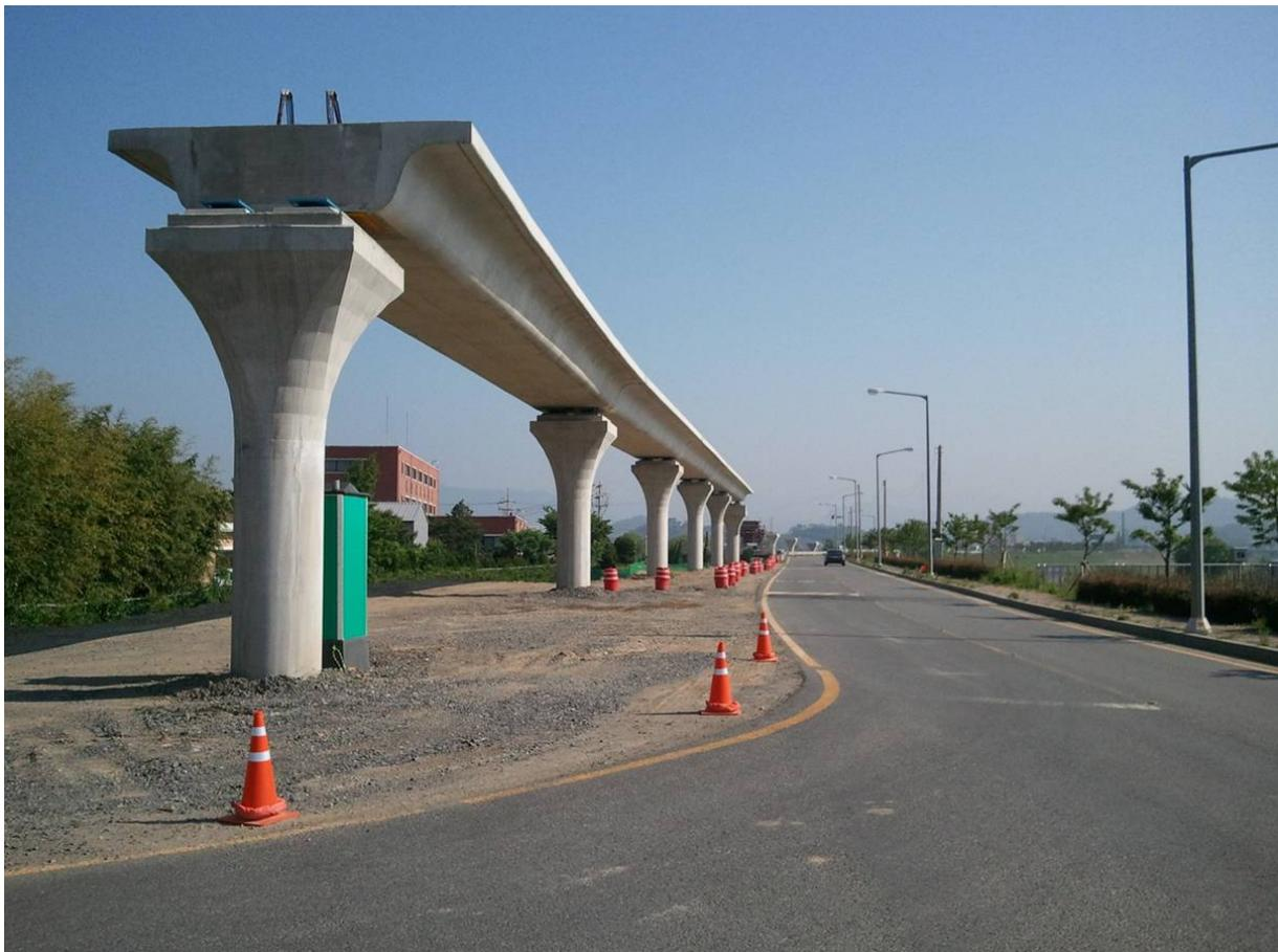
**Figure 6.** Concrete track consisting of concrete pillars and concrete girders being built at site in Suncheon.
