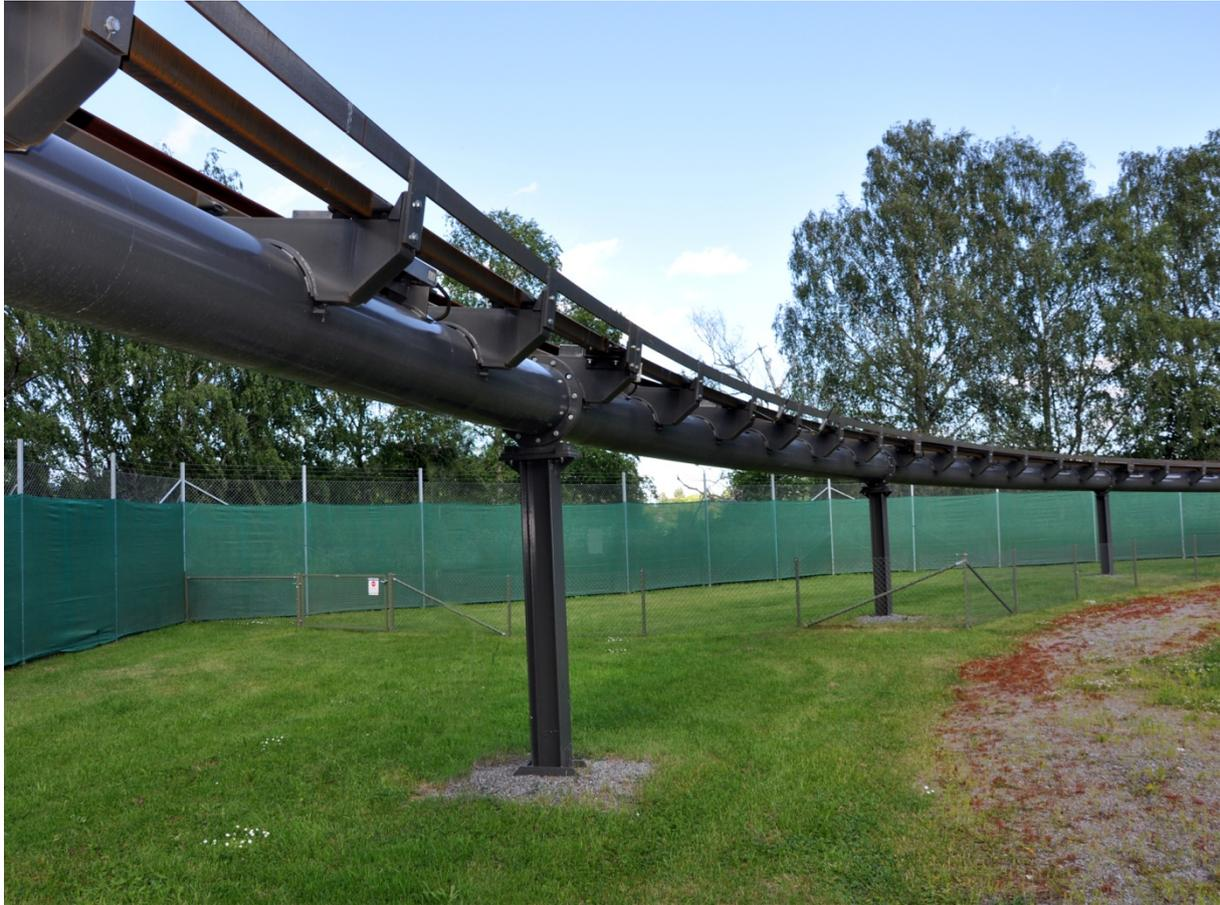
**Figure 7.** Steel track with concrete foundation at Uppsala test site.
